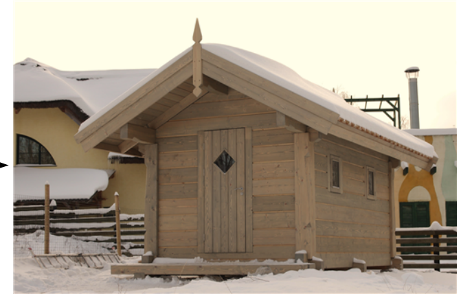
3RADI log wall with massive stud corner joint (wall do not settles at all)
